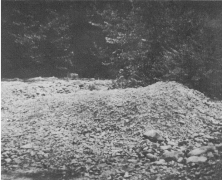
Figure 6. About 50 feet upstream of the railway bridge lies this large pile of gravel and cobbles left by past storm water discharges. The debris causes the stream channel volume to continuously decrease after each high water flow, thereby increasing the flood damage potential of successive high flows.
