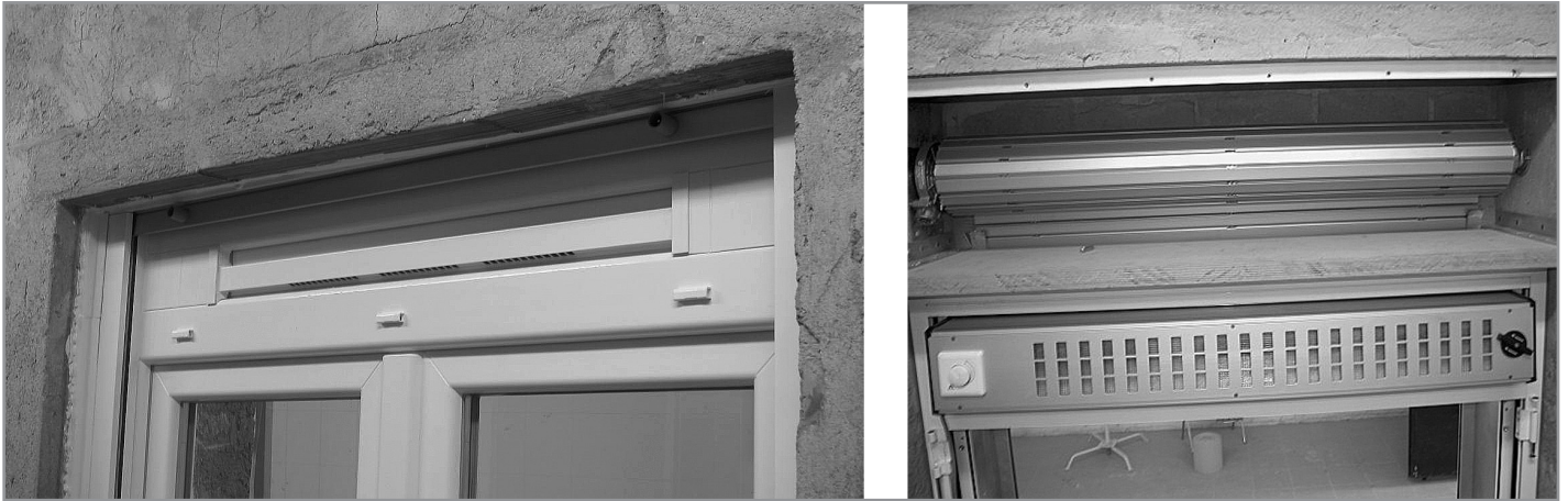
Figure 4. High Sound Insulation Ventilating Windows with rolling shutter boxes:
